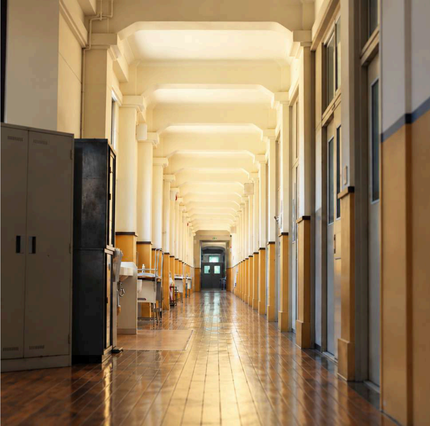
In the 1930s extension, moulded column heads and haunched beams create a high, colonnade-like corridor. The consistent treatment of walls and woodwork reinforces its long rhythmic perspective.
