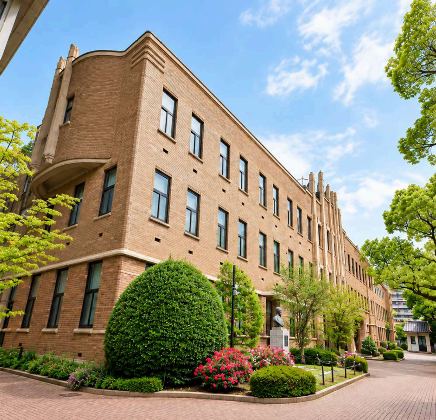
The exterior is faced with scratch tiles in subtly different tones, darker at the base and lighter above. Rounded corners soften the massing, while shadows on the textured tiles give the facade its calm character.
