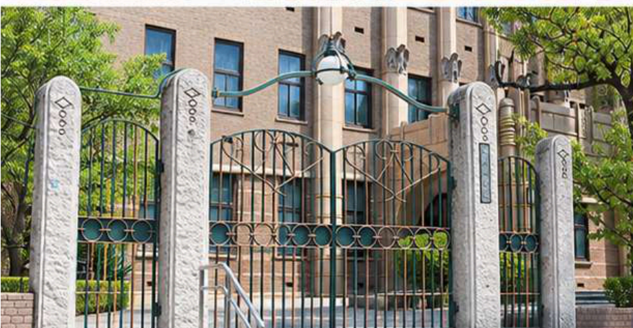
Former Main Gate, completed around 1929: four granite pillars frame the main and side gates across a width of about 6.4 m. The iron arch and lamp were conceived as a symbolic school entrance, and the basic composition survives today.
